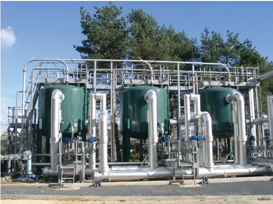
c. Granular ferric hydroxide adsorption plant, Severn-Trent Water, United Kingdom
