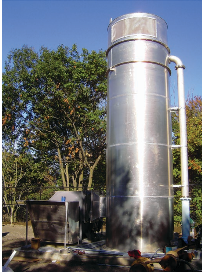
PHOTO 6.2. Example of an Air Stripping Column for VOC Removal
